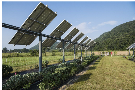
Photo credit: Dennis Schroeder/NREL
